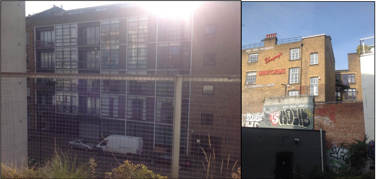
Image 5: View of adjoining buildings to the rear of the site.
